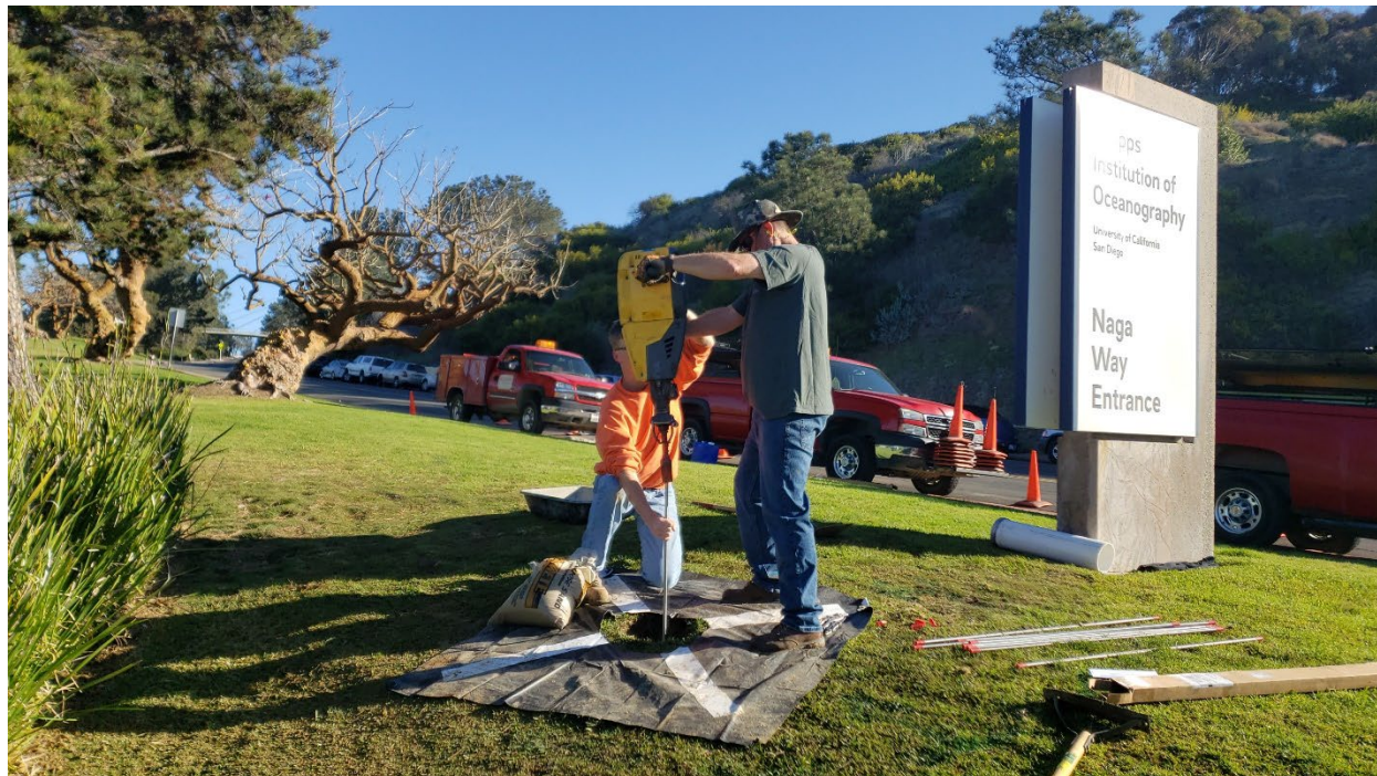
Figure 11. Installing new bench mark
