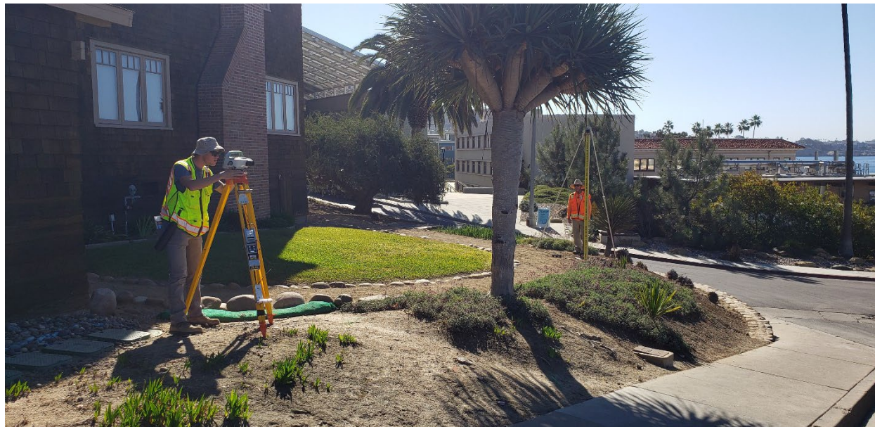
Figure 12. Surveying recently installed bench marks
