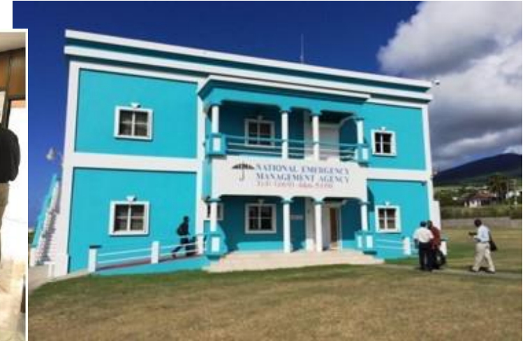
St. Kitts Emergency Operations Center
