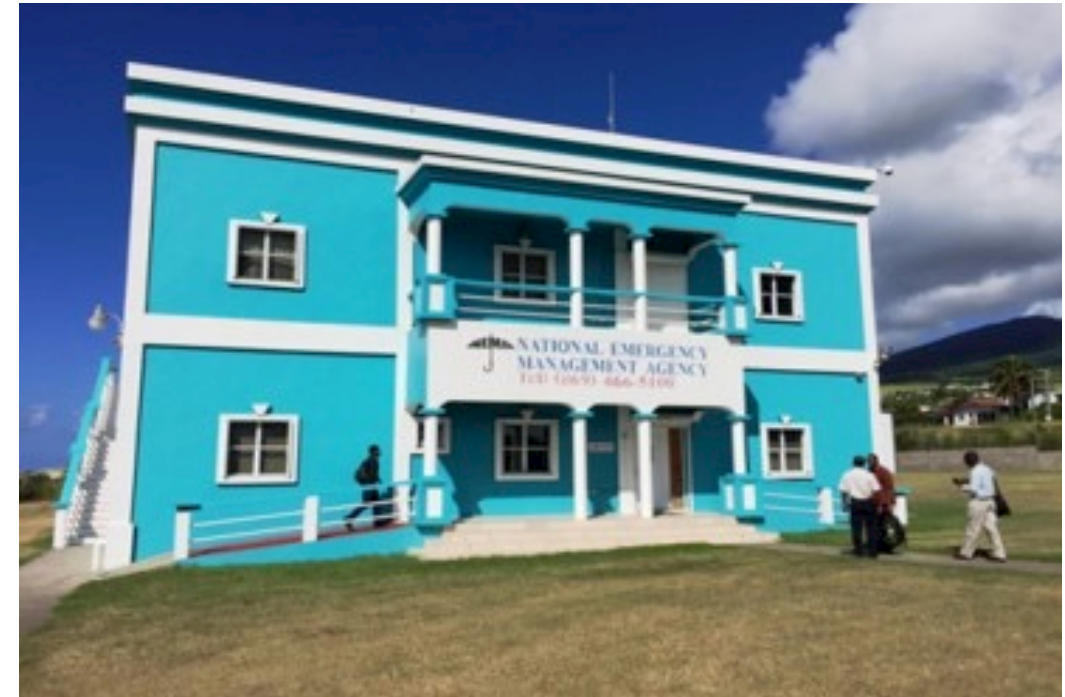
St. Kitts Emergency Operations Center
