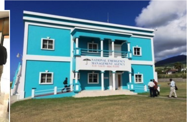
St. Kitts Emergency Operations Center
