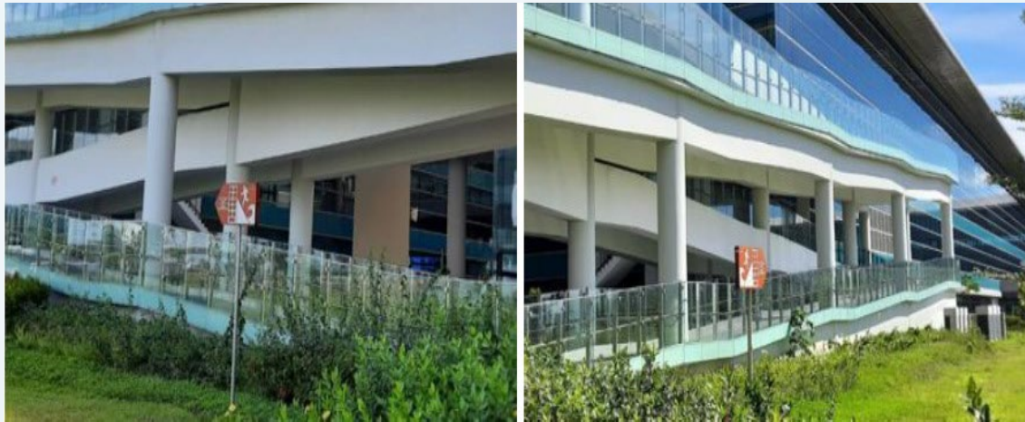
Evacuation shelter for tsunami in the YIA that also used by the community surrounding as the evacuation place
