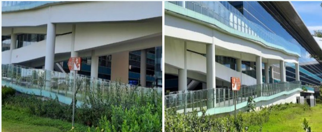
Evacuation shelter for tsunami in the YIA that also used by the community surrounding as the evacuation place
