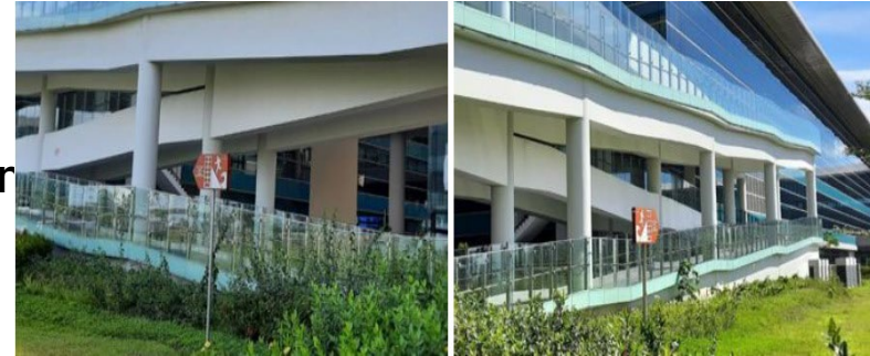
Evacuation shelter for tsunami in the Yogyakarta International Airport (YIA) that also used by the community surrounding as the evacuation place
