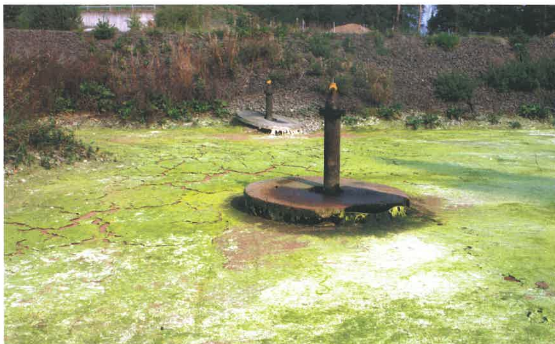
Fig. 2. The infiltration ponds at H ssleholm Water Works, Southern Sweden, have been clogged by Microcystis botrys , being present in the raw water. (Photo: Annadotter).
