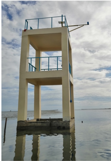
Installation of ultrasonic sensor and wet sensors (3m, 5m and 8m) at Prieto Diaz, Sorsogon Sea Level Station
