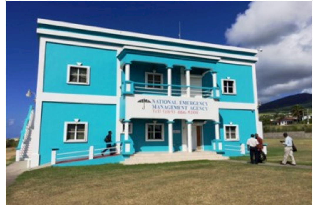
St. Kitts Emergency Operations Center
