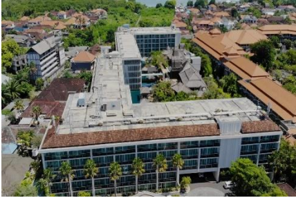
Hotel Roof Top for Vertical Evacuation
