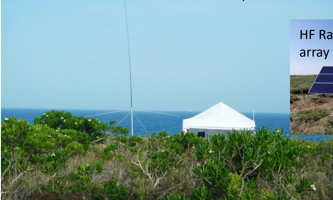
HF Radar on uninhabited Mona Island, Puerto Rico
