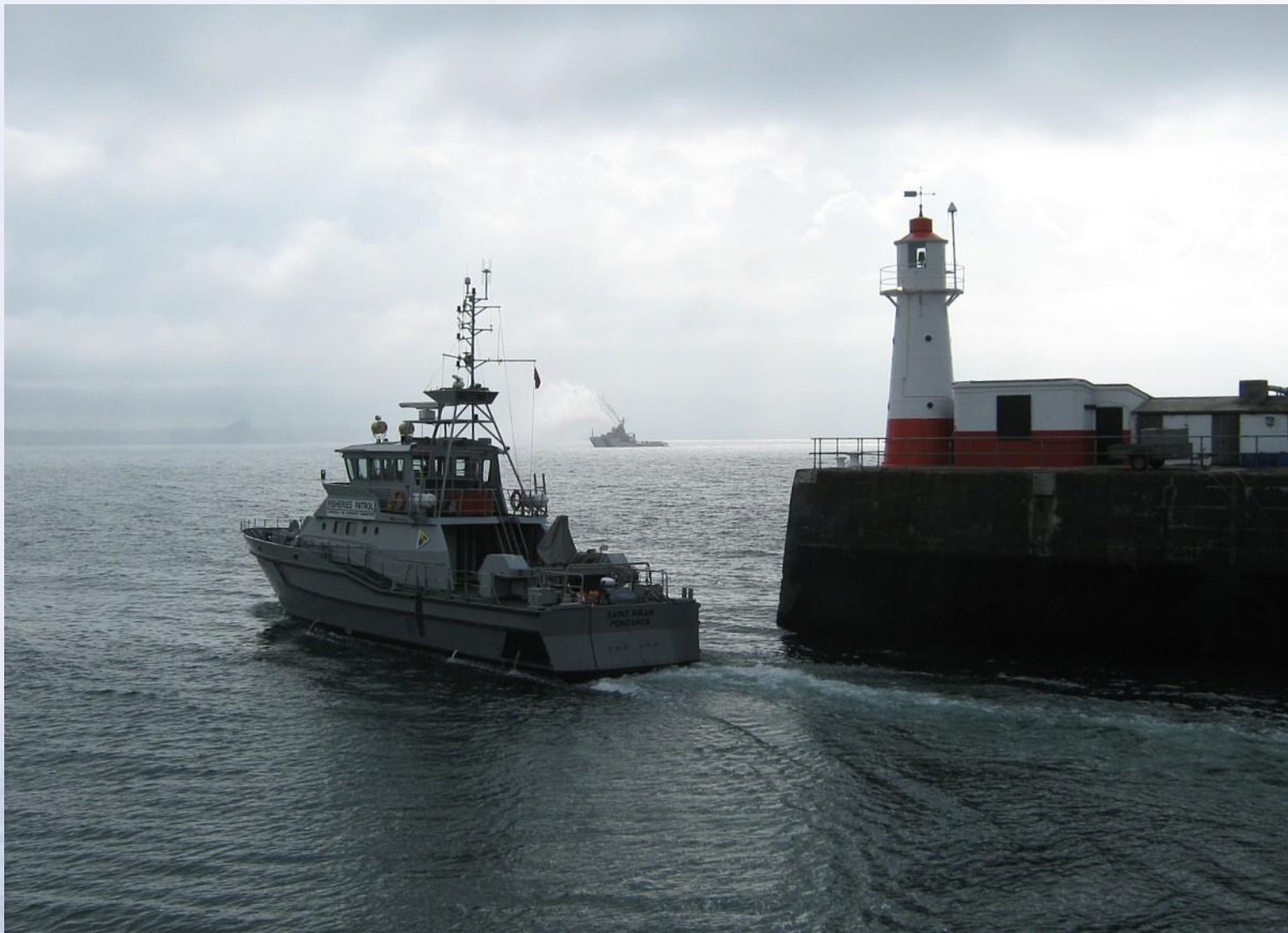
Newlyn tide gauge station, note the GPS antenna on the lighthouse used for GPS reflectometry test
